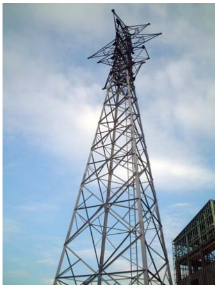
69KV 架空線進場鐵塔架設 69KV Over Head Receiving Tower installation
