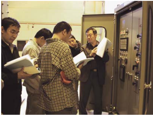
變電站教育訓練 Equipment Training
