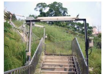
逃生梯照明工程 Emergency Lighting Fixture Installation
