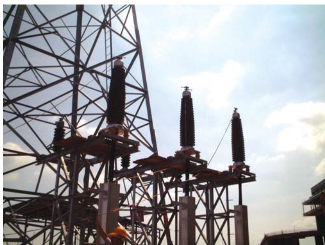
69KV 氣中電纜頭安裝 69KV Cable End Bushing installation
